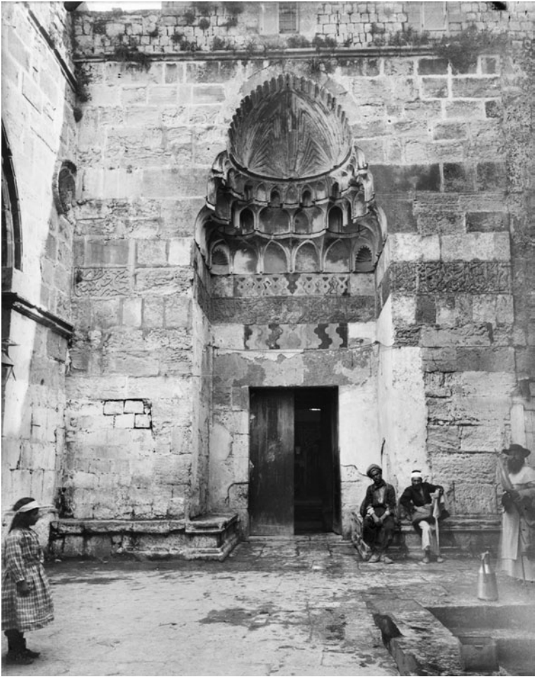
▲ Recessed entrance with mukarnas of the C14 theological school built by the Mamluk viceroy of Syria Saif al-Din Tankiz.
